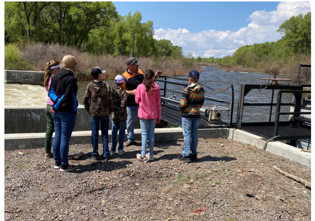
Nathan Coombs explains how an automated headgate helps to administer water.
